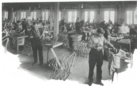
Frame building requires many careful, painstaking operations
